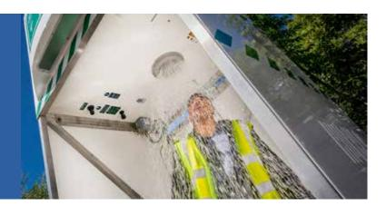
The most widely accepted international standard for safety showers and eye/face wash equipment, ANSI Z358.1-2014 specifies a tepid water supply to the shower, vital to ensuring worker safety.
